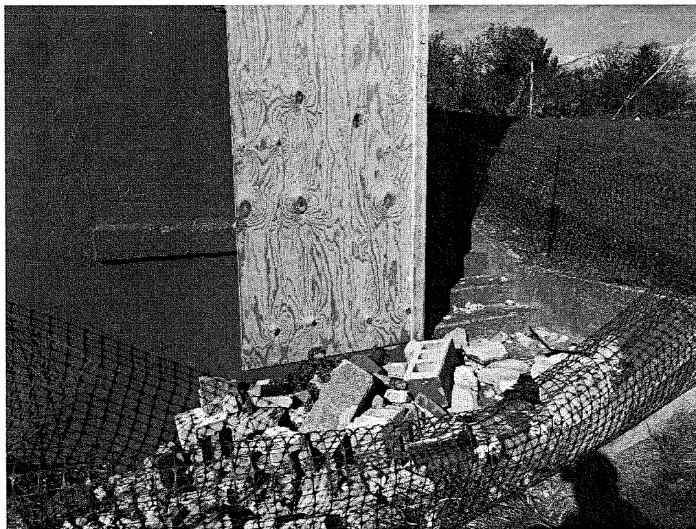
Exterior: Non-asbestos containing wall block, wall grout, brick, brick grout and red grout.
