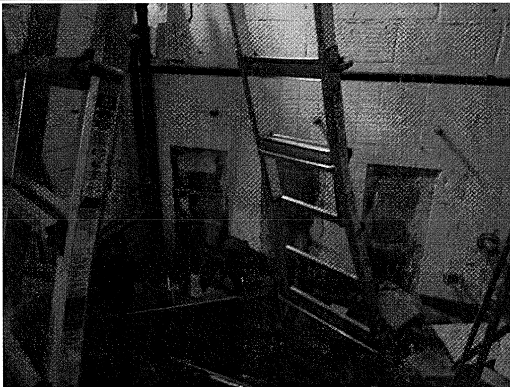
Ground Level: Non-asbestos containing black, white wall tile and grout.
