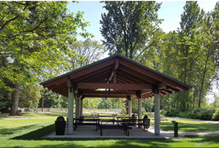
LARGE PICNIC SHELTER
