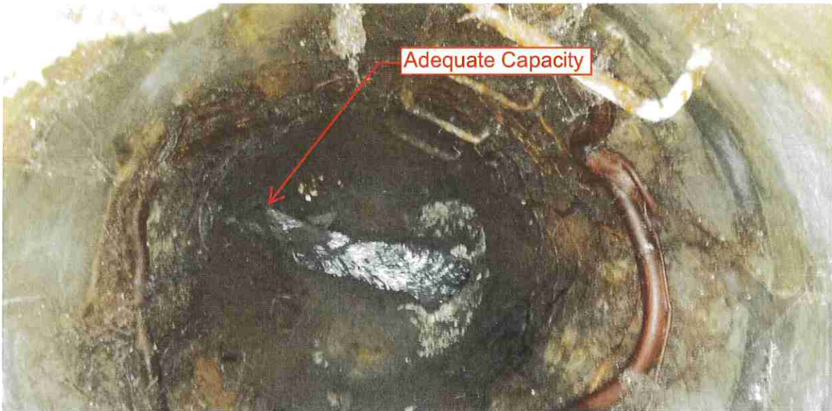
Manhole 54 B – Adequate Capacity
