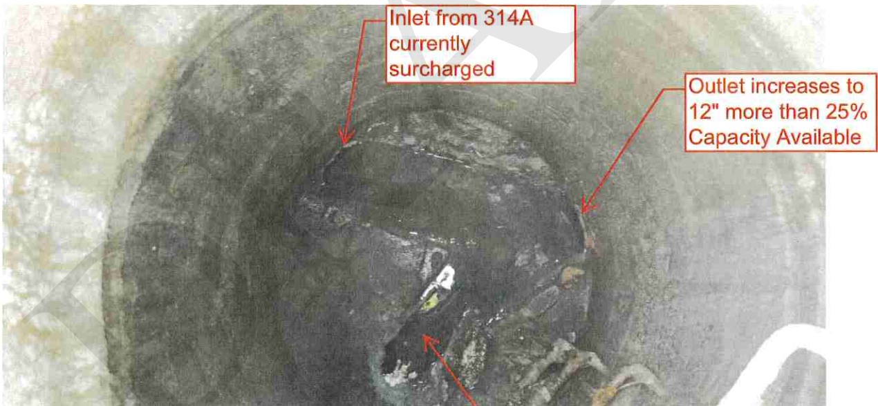
Manhole 314 – Adequate Capacity pipe sizes increase to 12"
