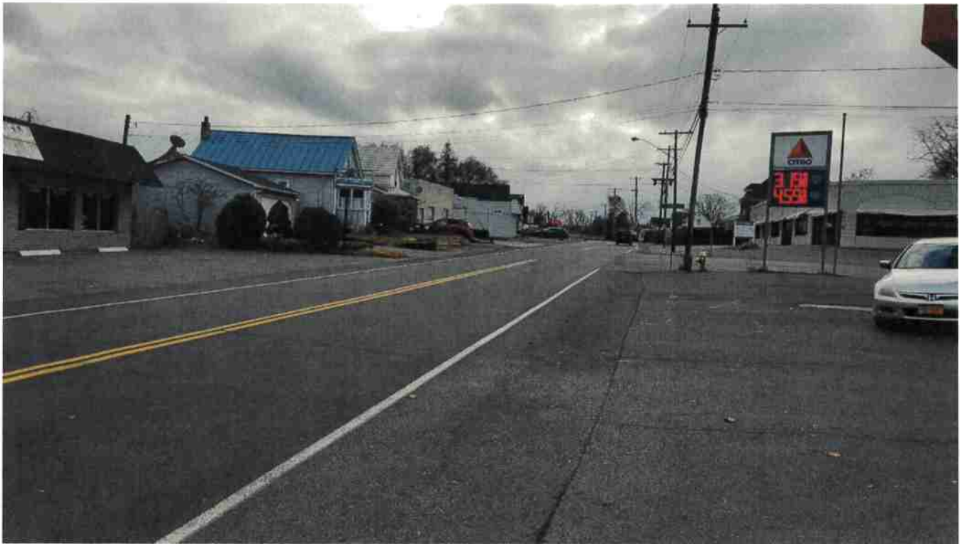
Figure 32: Example of Poor Access Management in the Study Area Image Source: JMT
