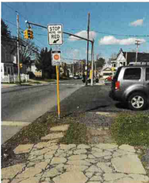
Figure 33: Existing Bus Stop in Study Area Image Source: JMT
