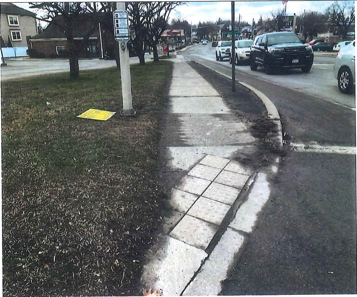
Photo 3 Example of Rating 4
