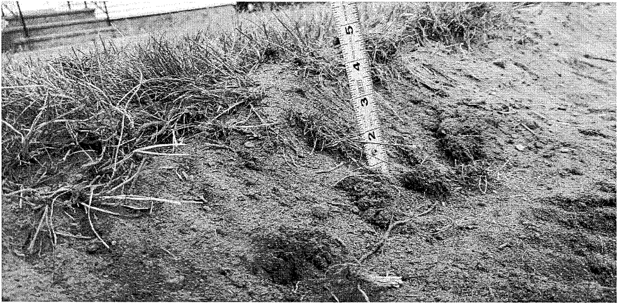
Excavation depth at #269 Princetown Road where transitions to existing lawn.
