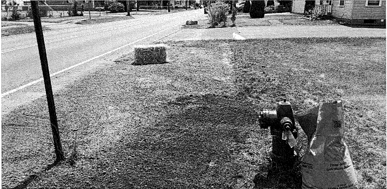
Grading of topsoil prior to seeding and mulching at #309 Princetown Road.
