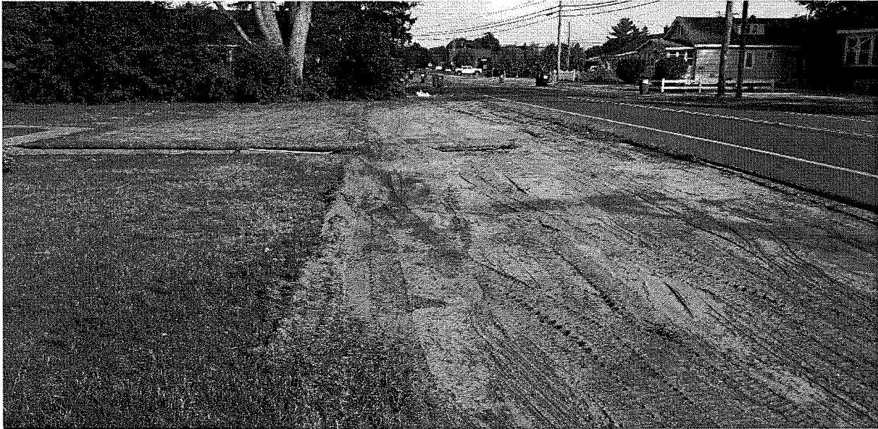
Rough grading of #269 Princetown Road.
