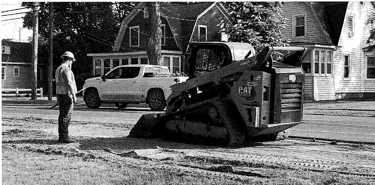
Rough grading of #269 Princetown Road.
