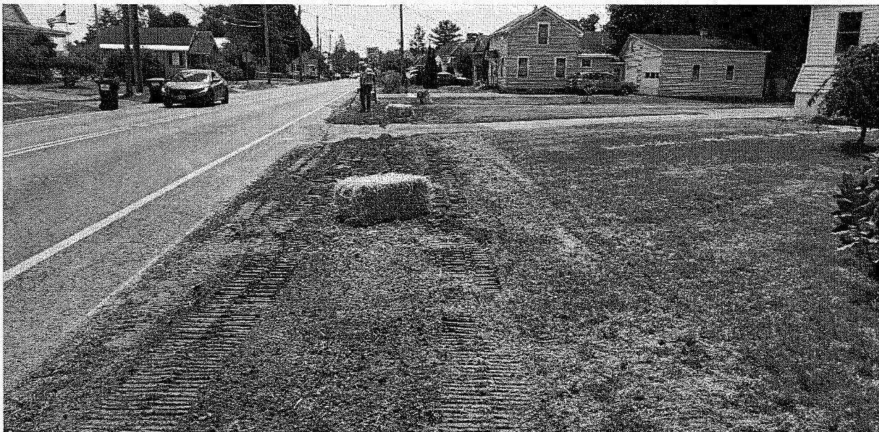
Grading of topsoil and stone removal at #305 Princetown Road.
