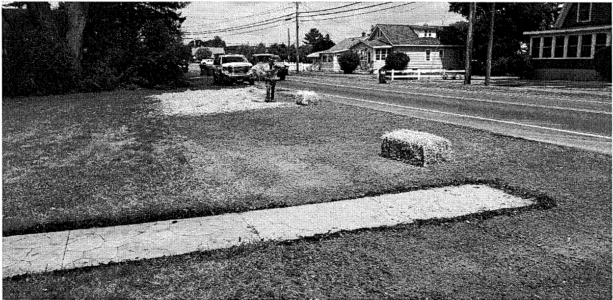
Topsoil, seeding and mulch placement at #269 Princetown Road. Lawn graded to drain away from the sidewalk to prevent potential ponding.
