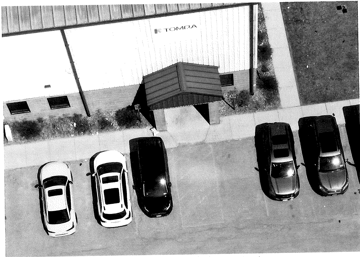
Existing ADA parking with signage at entry
