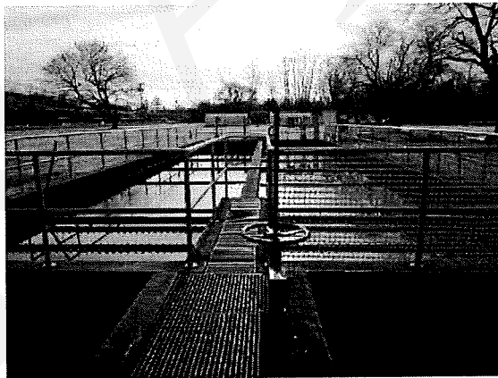
Figure 3-7: Secondary Clarifiers
