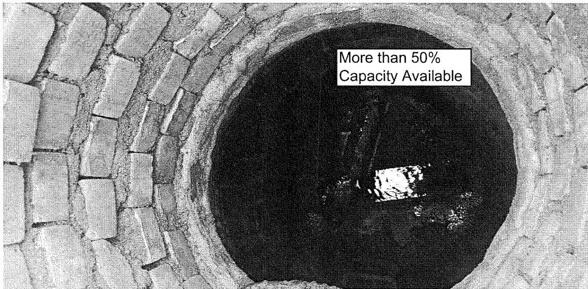
Manhole 312 - Adequate Capacity
