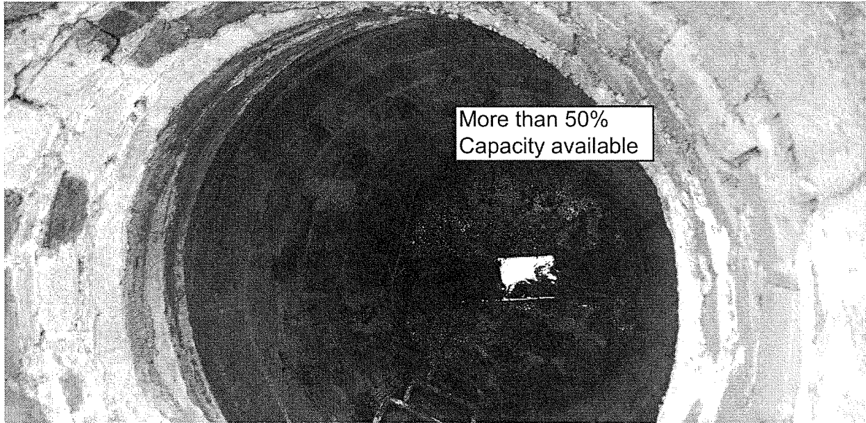
Manhole 312 A – Adequate Capacity
