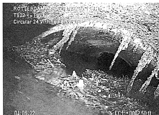
Figure 2: Root Intrusion
