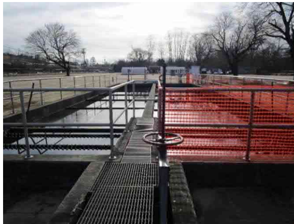
Figure 3-7: Secondary Clarifiers
