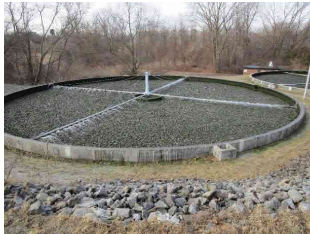
Figure 3-6: Trickling Filters
