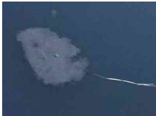
Figure 3-8: Floating Sludge in Chlorine Contact Tank
