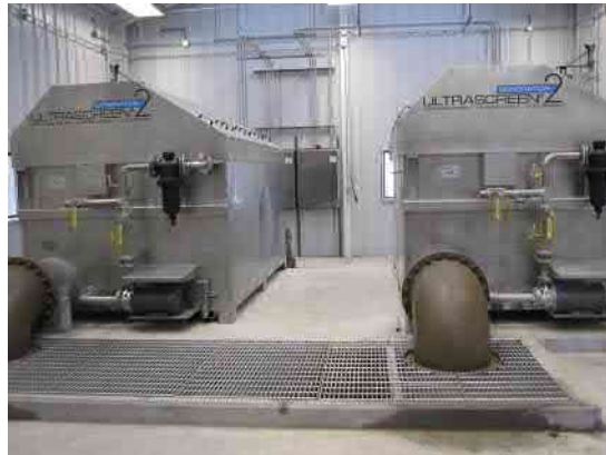
Figure 5-2: Disk Filter Installation
